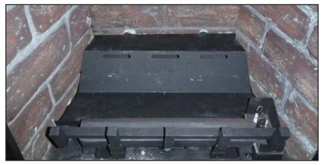
Figure 41. Empty firebox with grate and locator pins.
