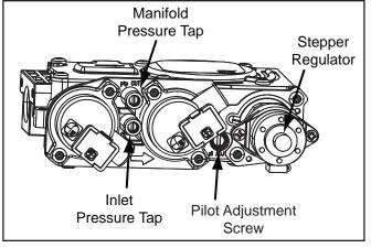
Figure 39: Fully Labeled Gas Valve. See Dexen User Manual for S20ID valve details
